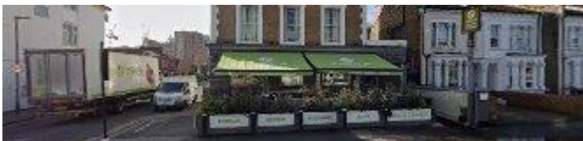
Front elevation facing West
